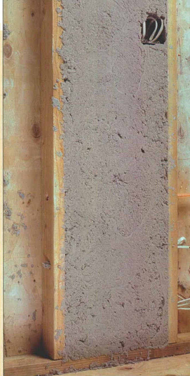
3. Dense-packed to R-3.5 per in., and also air-sealed.
