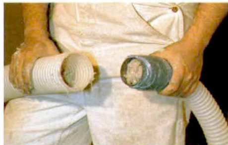
Clogs occur where the hoses reduce in size. Disassembling the joint and blowing the blockage from the large hose clears both of the pieces.
