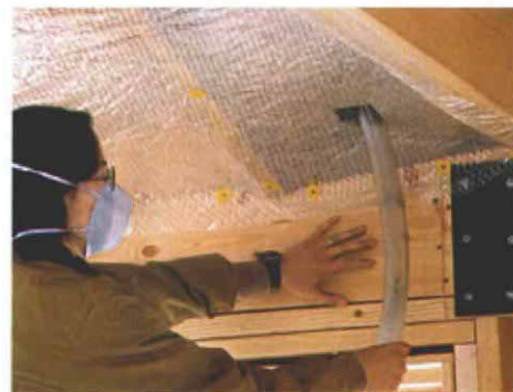
When rigid sheathing isn't practical, membranes can work. They won't hold the density that sheathing can, but membranes seal irregular areas more easily.
